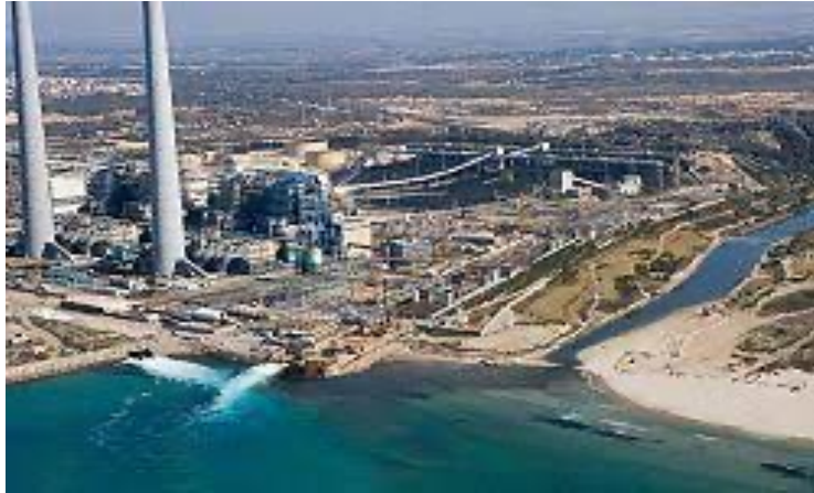
5 desalination plants that provide in total 850 MCM/year First plan operation: 2008
